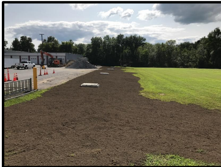
Grading Around Sanitary Access Pits
